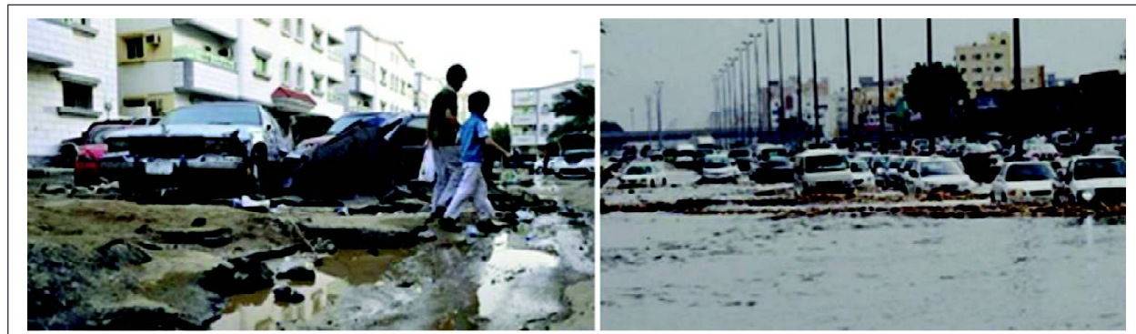
Figure 2: The engineered stormwater infrastructure fails to cope and adapt to excessive rain rates.
