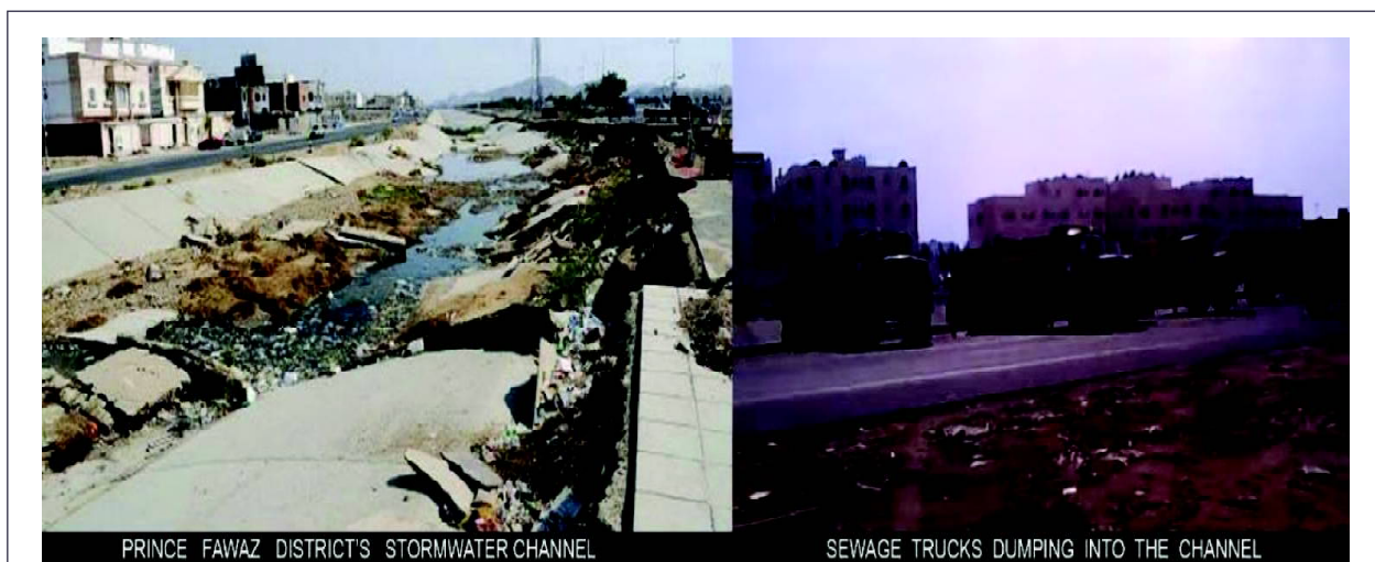
Figure 4: Dumping black-water and solid waste at the drainage channel of Prince Fawaz district, Jeddah city.
