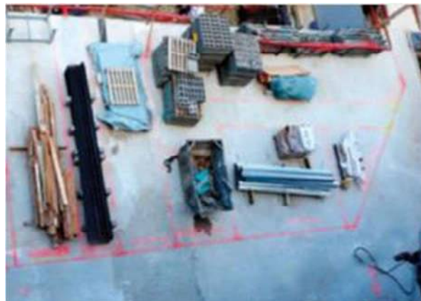
Figure 5: Tape to Delineate Material Lay-Down
