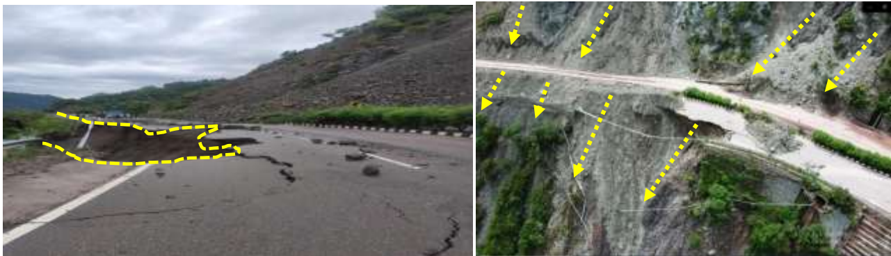
Figure 1 NH-05 Road Affected Near Koti area (Between Parwanoo to Sanwari) in 2023. (Source: HPSDMA and analyzed by the author.)
